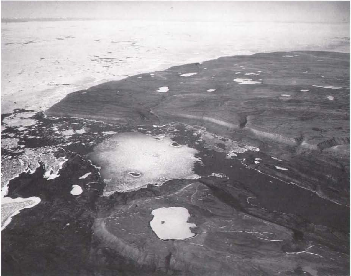
Fig. 1. The south-eastern margin of the Franklinian Basin in Greenland. Pale weathering Cambrian siliciclastic and carbonate sediments overlying darker Precambrian crystalline basement at Marshall Bugt, Inglefield Land. Aerial photograph looking north across Nares Strait toward Ellesmere Island. Copyright, Kort- og Matrikelstyrelsen, Denmark.
