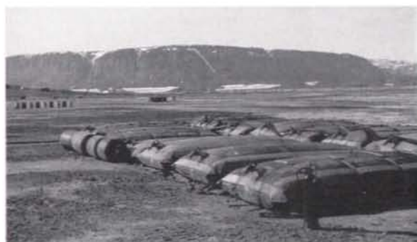
Fig. 9. Rubber bladder tanks for aviation fuel, each with a capacity of 3500 l, at Kap Moltke.
