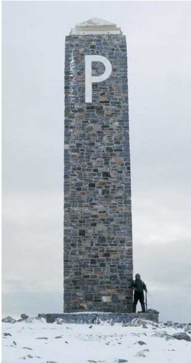
Fig. 13. Pearys Mindevarde on the plateau at Kap York. This three-sided monument from 1932 is c. 30 m high. Apart from the marble forming the letter 'P', the column is built of rocks of the Kap York meta-igneous complex collected and quarried nearby. The mosaic is made up of blocks varying from dark grey (gabbro/amphibolite) to buff (granodiorite/granite), with the predominant rock being a grey, mesocratic tonalite/quartz diorite. Avatak Henson stands guard, 16 September 1974.
