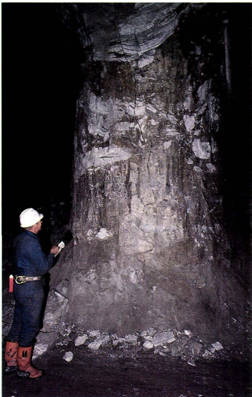
Fig. 2. Typical ore left in pillar in the Cover zone of the Black Angel mine. Fractures indicate that the maximum load-bearing capacity of the pillar has been exceeded. The ore consists of sphalerite, galena and pyrite. White marble rafts and inclusions are conspicuous in the upper part of the pillar.
